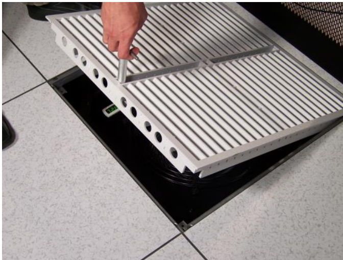
Figure 20 - Installation of DirectAire ® Panel
