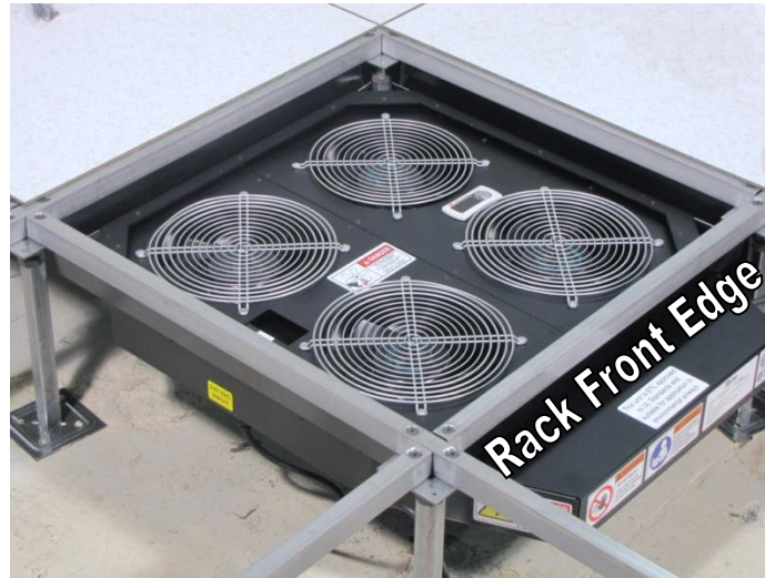
Figure 7 - PowerAire® Quad Unit Installed on hangers in correct orientation
