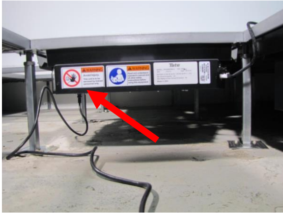
Figure 15- Connecting power to the unit
