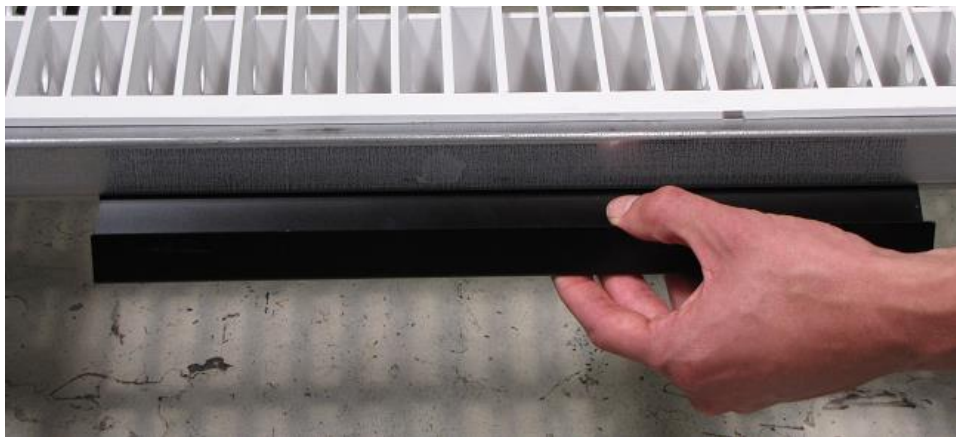
Figure 3 - Insert hanger into roll form opening and catch the top angle inside the stringer
