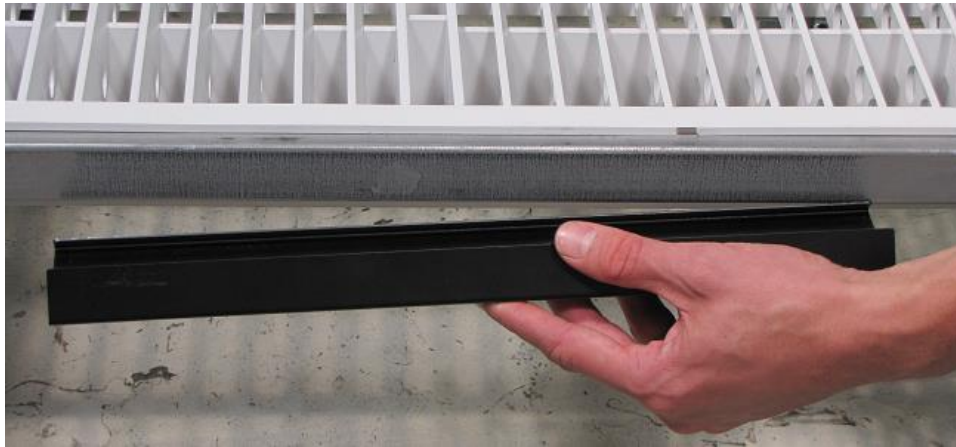
Figure 2 –Position hanger parallel to the floor with short angled edge aligned to opening in roll form stringer
