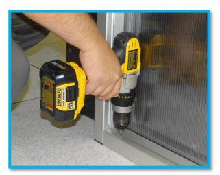
10. On the right hand side, drill the side door post to the floor. Drill behind the post frame.
