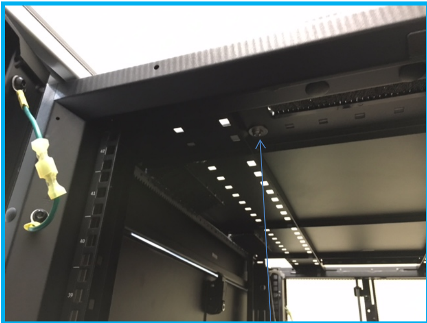
Bolt and Washer bolted into T-bolt
