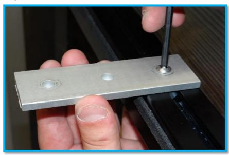
18. Secure the header to the rack with the server mounting hardware. We recommend thru bolting the door to the server.
