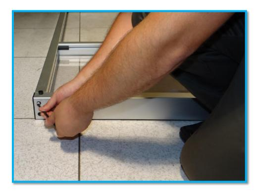
11. Place end caps on the header once the screws have been secured.
