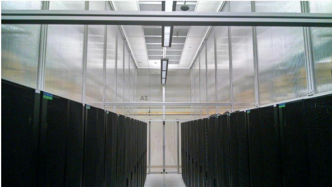
Hard Partitions suspended from above as part of hot aisle containment; note ceiling return grilles
