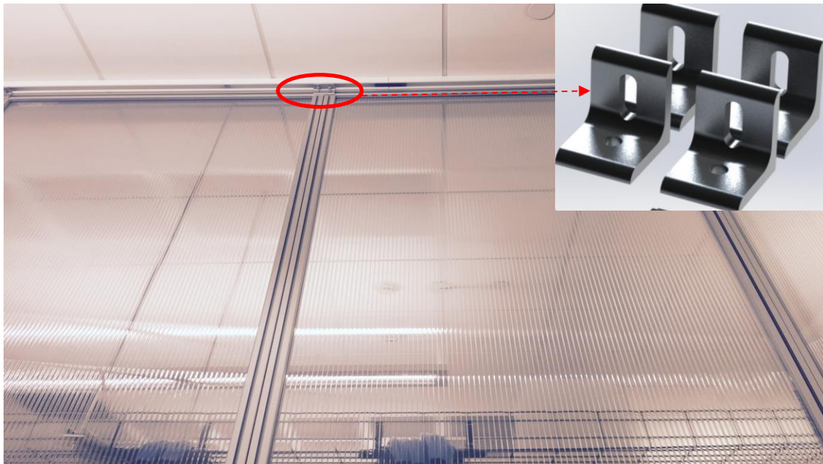
In this installation, angle brackets are used to secure the hard partitions to their above support member
